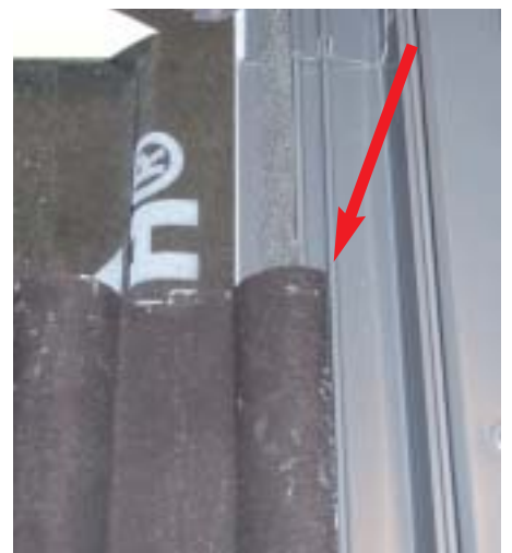
closing of roof covering to the high rib of edging
