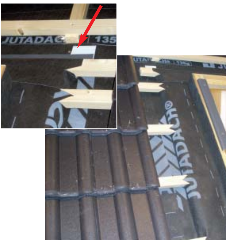
meeting of hydroisolation foil and placing of drain channel
